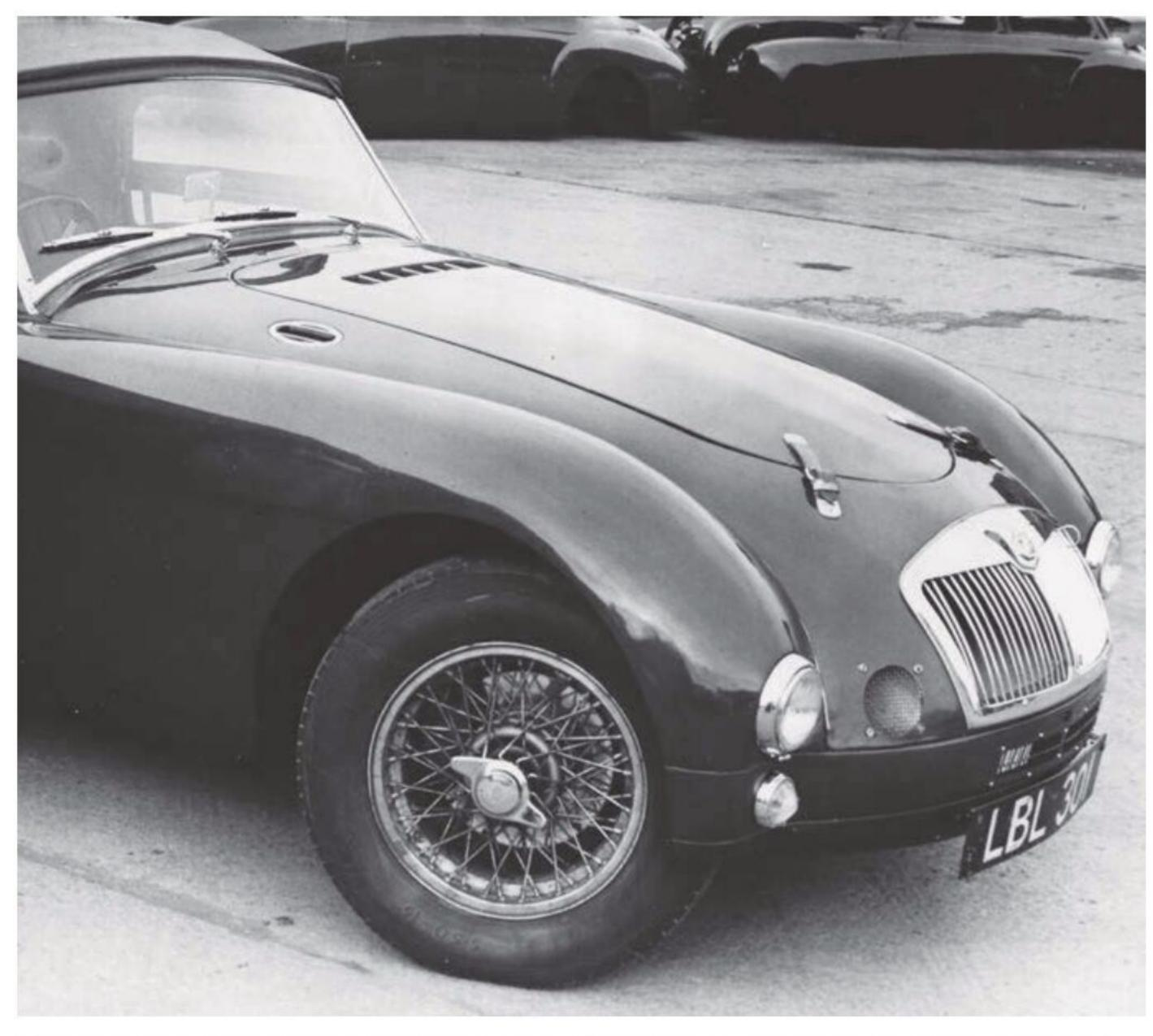
This was how Abingdon re-prepared an EX182 Le Mans prototype, with low-mounted headlamps, to see if the aerodynamics were improved.
